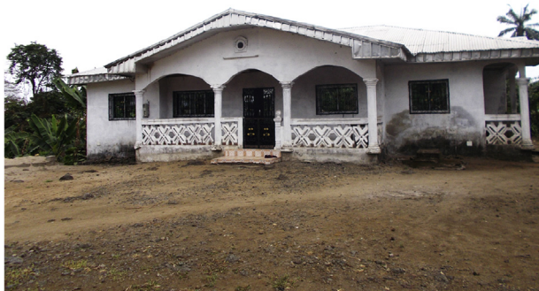
Fig. 9. Example of a block house considered suitable for LPG use (P4, M, age 47, Rural, Income 1).
